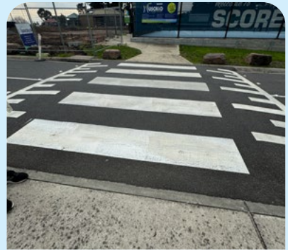
Wombat crossing improves safety and connectivity between footpaths. SV
