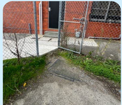
Step at end of footpath through gate difficult for PMDs to use. SV
