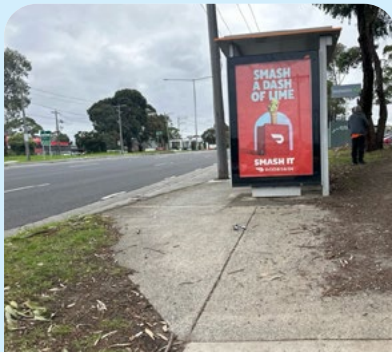
Footpath does not align with the desire line. SV
