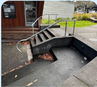
Stairs have rail and tactile markers. TBT
