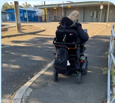
Narrow sloping footpath with no ramp makes train station inaccessible. FTG
