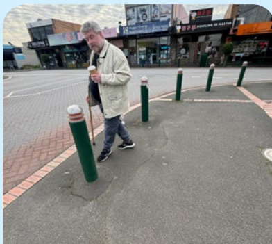
Bollards are a potential tripping hazard if there is no contrast painting. SV
