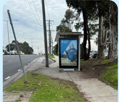
Bus stop infrastructure obstructs footpath. SV
