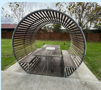
Seating cover does not extend so PMDs would not be protected. SV
