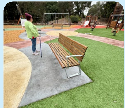
Bench installed on concrete pad, has arm rests and is connected to footpath. RCC
