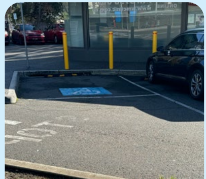
No shared zone, no ramp onto footpath, too short. WM
