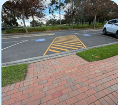
Accessible car parking located at footpath into park and has shared zone (but no bollard). Arboretum FTG
