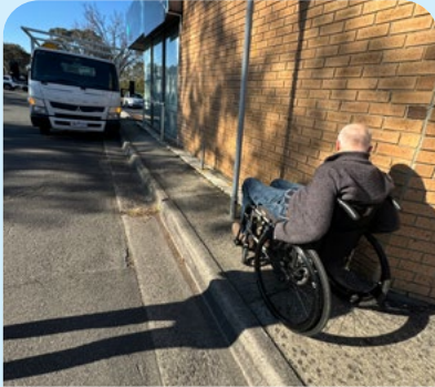
Sign post obstructs footpath. KF
