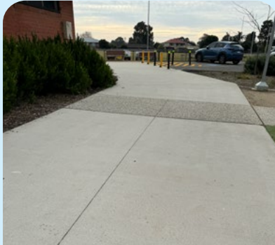
Wide pathway next to the accessible car parking space. SV
