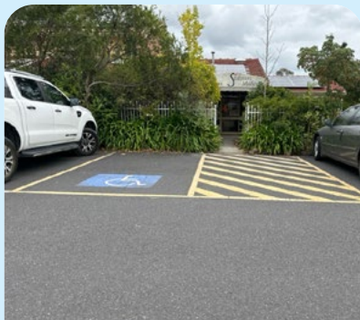
Bollard has not been provided in shared zone. SV
