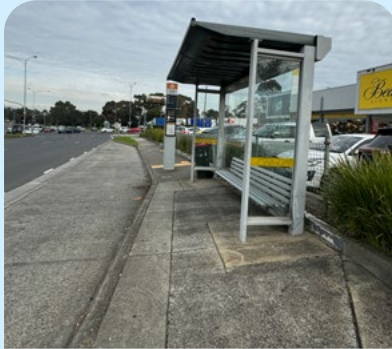
Bus stop infrastructure obstructs footpath. SV
