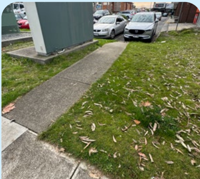
Footpath terminates and does not connect to anything. SV
