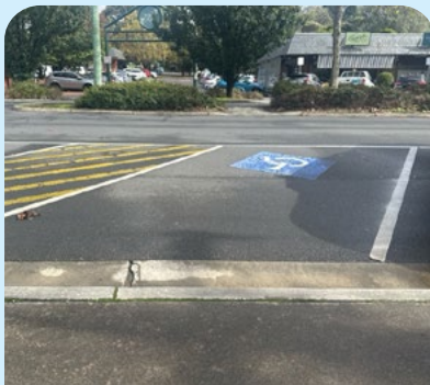
Dedicated accessible parking space line markings are not yellow. FTG
