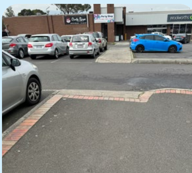
Steep pram ramp and not safe to cross. SV
