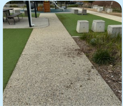
Wide footpath with good-quality surface. SV
