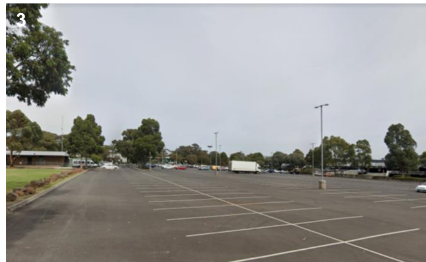
3 Existing Westfield-owned Carpark Consideration of the existing abutting car park and understanding its impact now and into the future.
