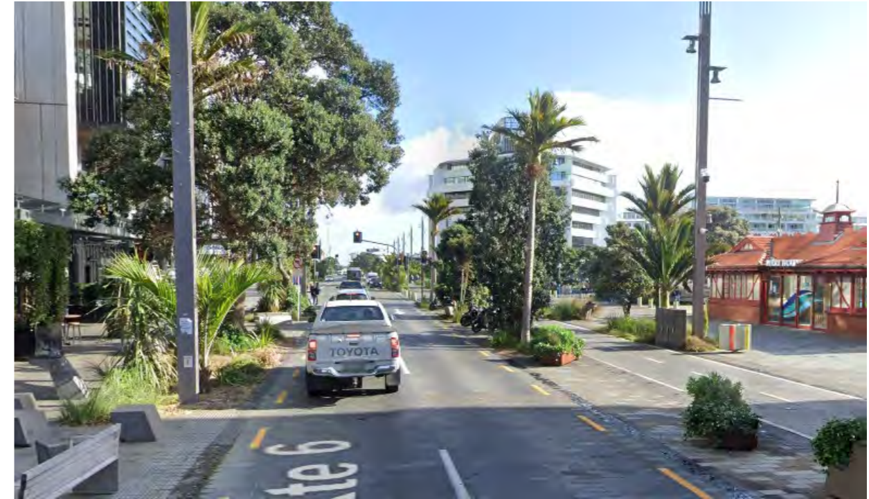
Figure 33: Dedicated two-way bicycle path with vehicular traffic on one side, Auckland, New Zealand
