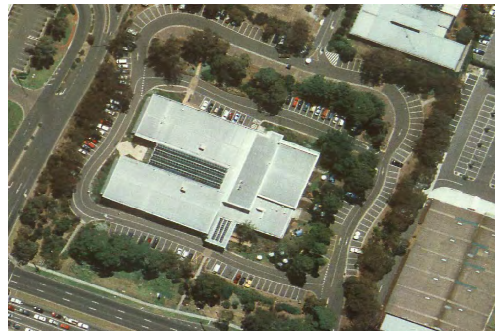
Figure 4: Aerial view of the Civic Centre building with completed atrium, 2001
